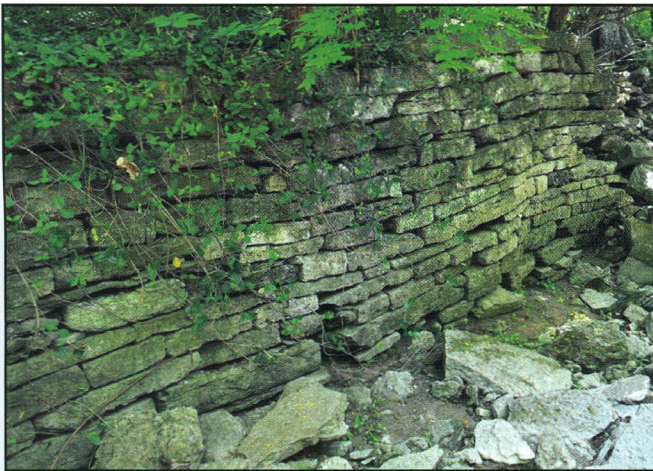
Dry-stacked fieldstone defines the side of the Mill Creek stream, near the house, and has survived well over the many years of rushing flood waters.
