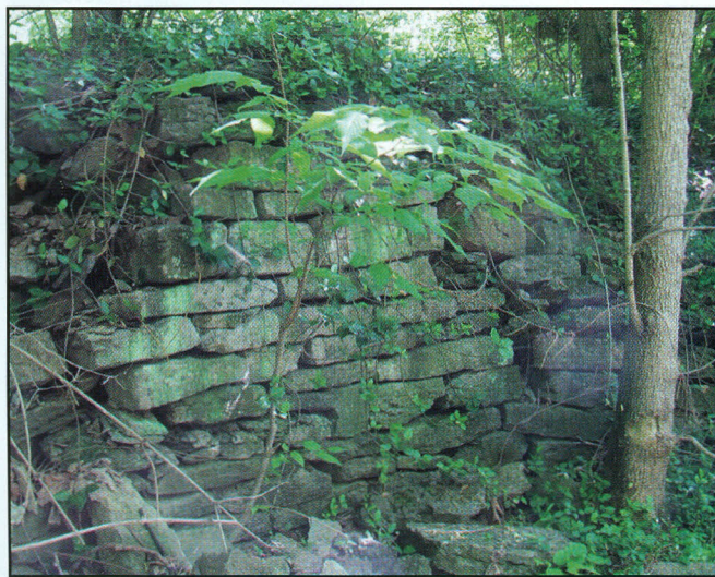
Here we see the dry-stacked stone suspension bridge abutment on the side of the branch of Mill Creek where the Lane house still stands. While the base of the pier remains in good order, the top level has deteriorated over time causing the loss of the anchor stones that held the cable support tripods.
